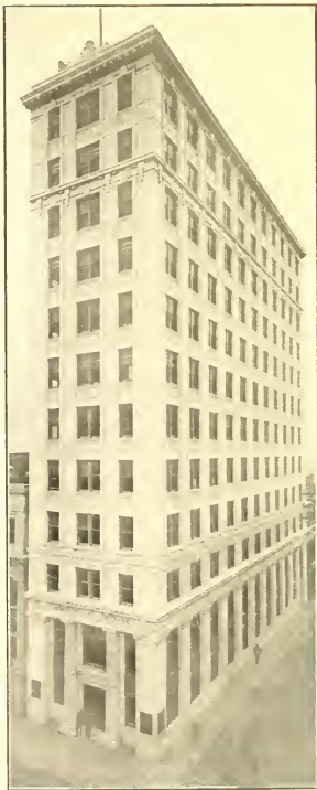
COMMERCIAL NATIONAL BANK BUILDING
